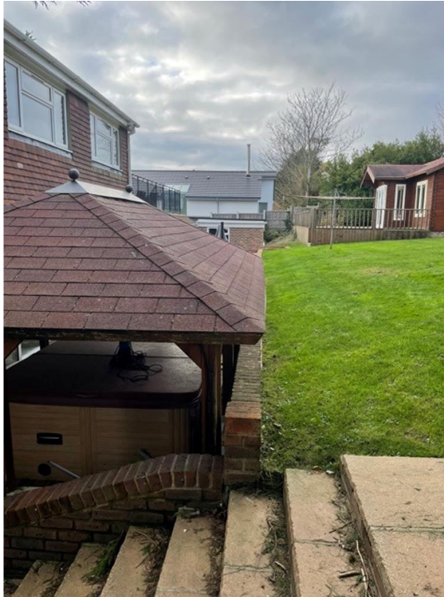
View looking west towards No. 35A
