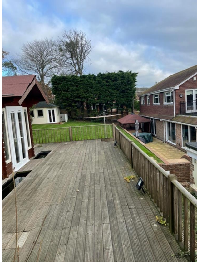
View looking east towards 2 Tree Tops Close
